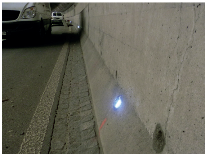
Tunnel Stephanshorn San Gallo
